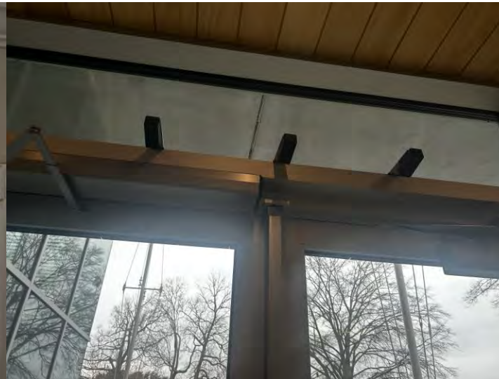
Kendeda Frame Material: Aluminum Type: Lip, about 2" thick, 1" deep
