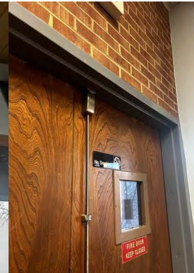
Weber Interior Frame Material: Coated Steel Type: Lip (Very Tiny < 0.1") Con: Coated Steel has weaker magnetic field
